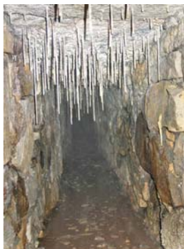
Passage downstream of entrance shaft
